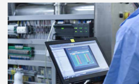
Equipment Assembly and Debugging
